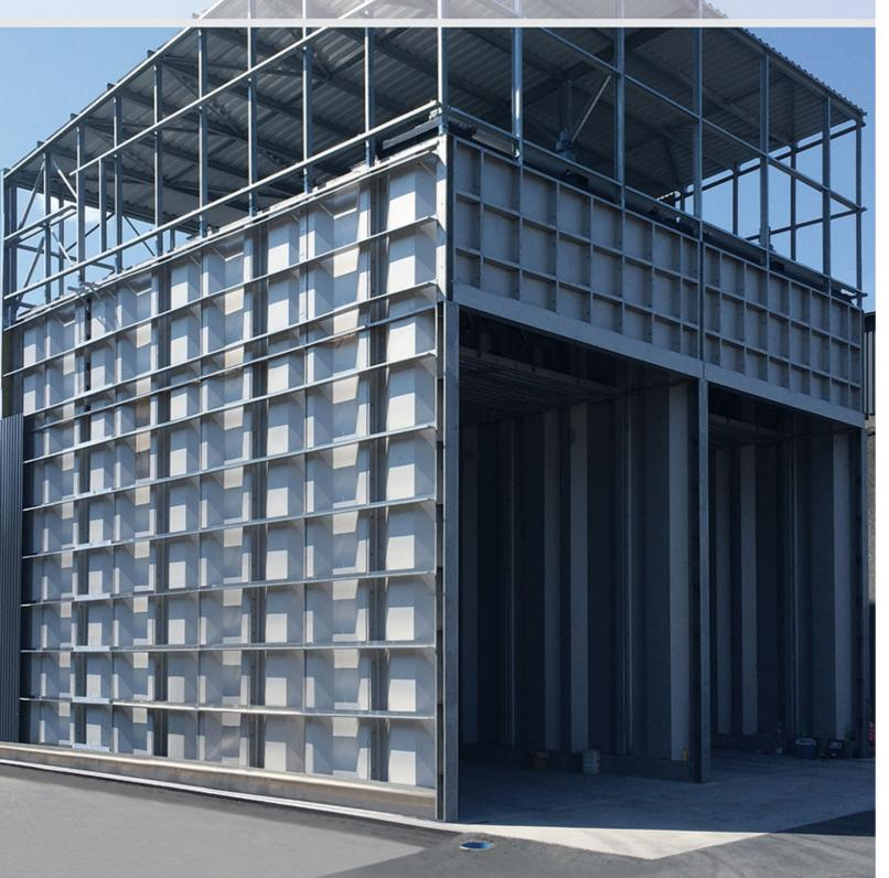
Therefore, as an Example, we are using only good quality Stainless Steel in Duplex Quality for our Framless Building Construction. Wall and Ceiling Panels are self-supporting and serves both as structure and climate shield. The High-Quality raw material is delivered directly from the Steel Mill
