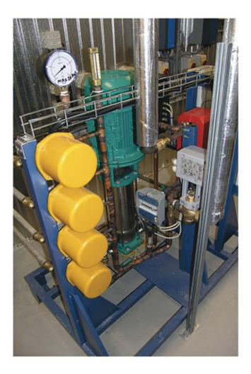
The high pressure pump is frequency controlled to conserve energy and provide the right volume of water at different stages in process. The soft start also reduces the pressure surge in the piping before and after the pump. In addition, the system that deliver the water fog has to have an unquestionable reliability. Through a clever and well thought out system we can ensure the water supply to the dryer, even if an accident should occur, stopping a pump or the flow through the heat exchanger.
