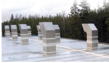
recovery unit itself uses a large-area counter-current flow system for ventilated and intake air. This system was specially developed to allow for the recuperation of heat in the lumber kiln. The heat recovery units of this type are dimensionally larger and structurally more complex than lamellar heat recovery units, however their system makes them the only truly effective heat recovery option that can be used for lumber kiln conditions.
