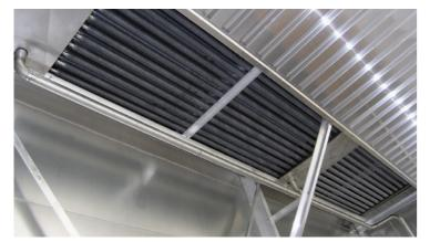
Our heating coils are made from stainless-steel pipes onto which an aluminium surface is rolled into the shape of ribs. The pipes lead into a collector that is connected to the supply and return pipes of the heating system. The heat output of the registers is proportioned for the maximum necessary heat output i.e. for the heating phase.
