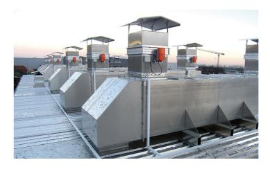
The air exchange system is made up of two rows of pipes in the ceiling of the kiln that draw in fresh, dry air, and release air saturated with evaporated water. These pipes are also manufactured from aluminium and are fitted with a regulating flap that is controlled automatically by a servo drive. The air exchange system may be connected to a heat recovery unit that allows for pre-heating of the intake air, conserving some of the heat energy. The heat
